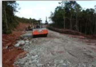
Reinforced existing 41km dirt road
