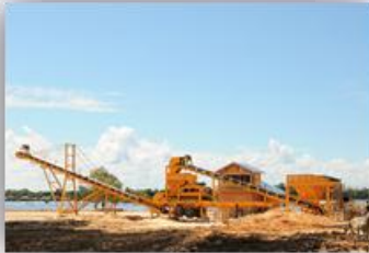
New jetty under construction
