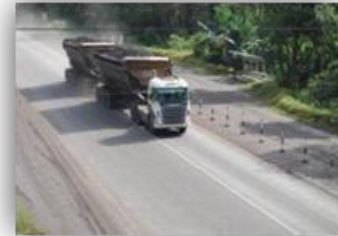
Upgrade existing 41 km dirt road to a new 35km tar road
