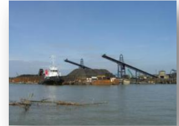
Enhance new jetty and loading facilities
