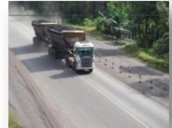
Upgrade to a new 35km tar road
