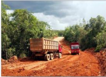
41km dirt road from coal mine to Telang baru jetty
