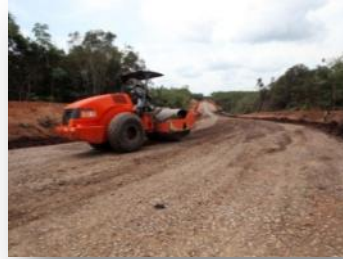
Reinforced existing 41km dirt road
