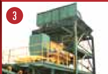
Coal Crushing and Stockpiling at Telang Baru Jetty
