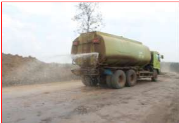
Regular road maintenance and widening
