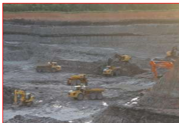
SEM Coal Mine: Pit 2 (Back fill in progress)
