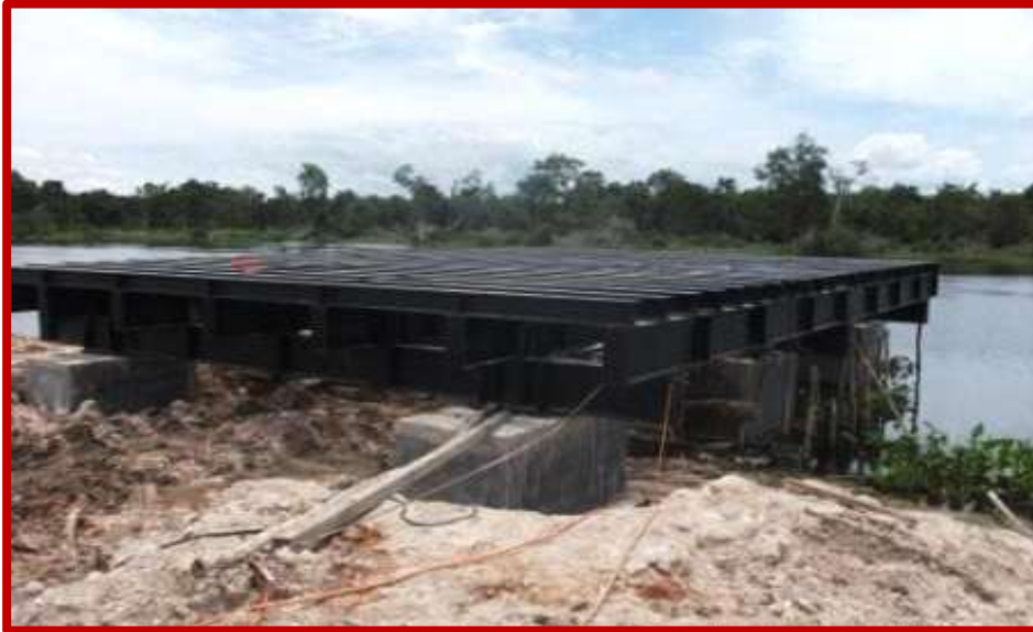
Construction of new loading port
