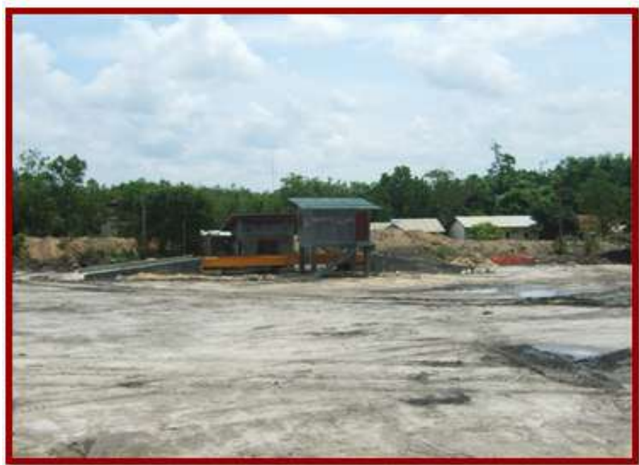
New weigh bridge
