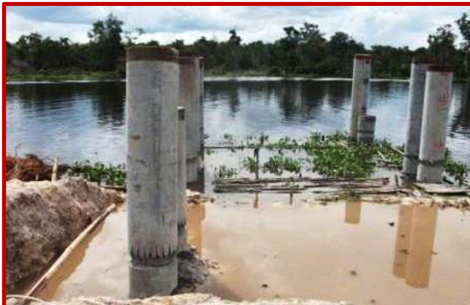
Piling works at new jetty
