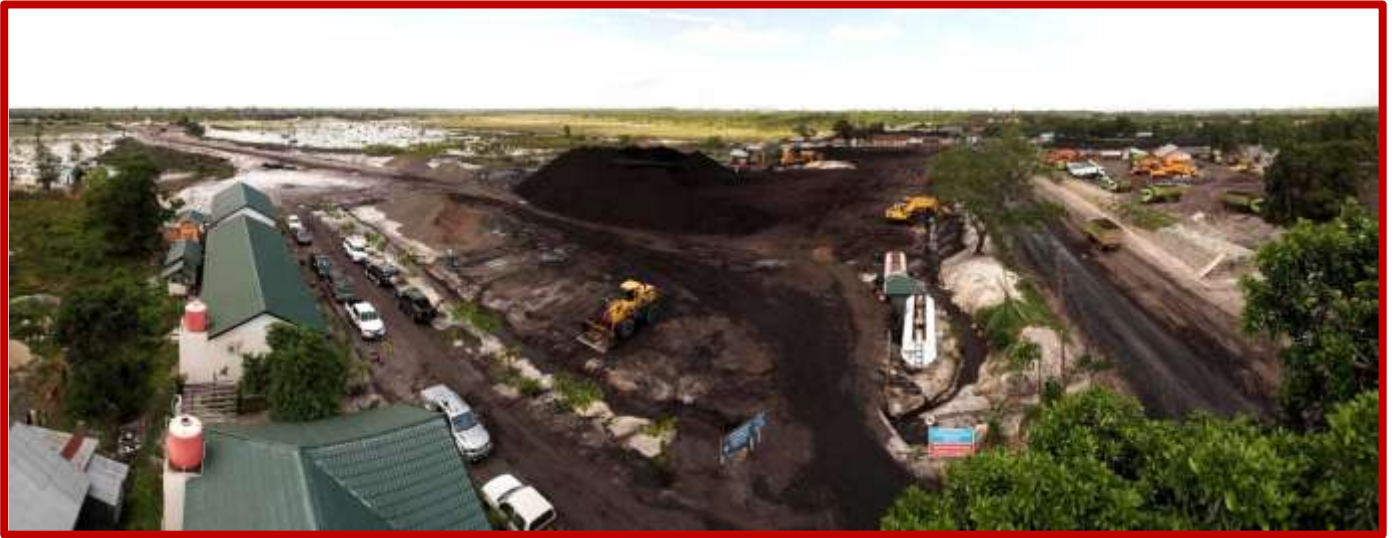
Existing stockpile and jetty (Panorama view)
