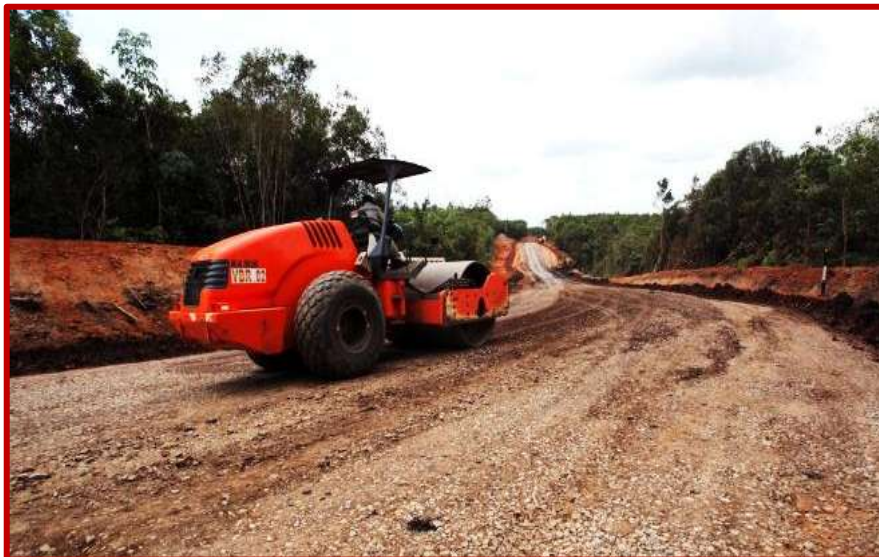
Regular road maintenance and widening
