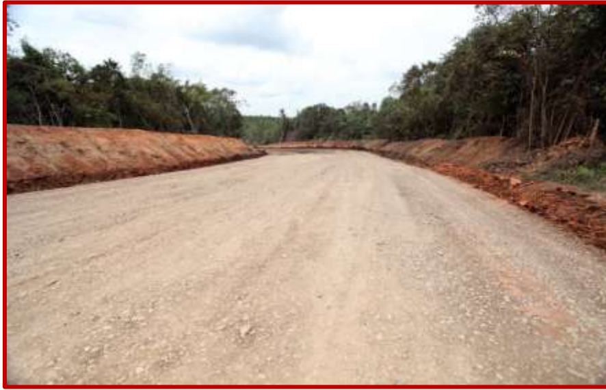
Regular road maintenance and widening
